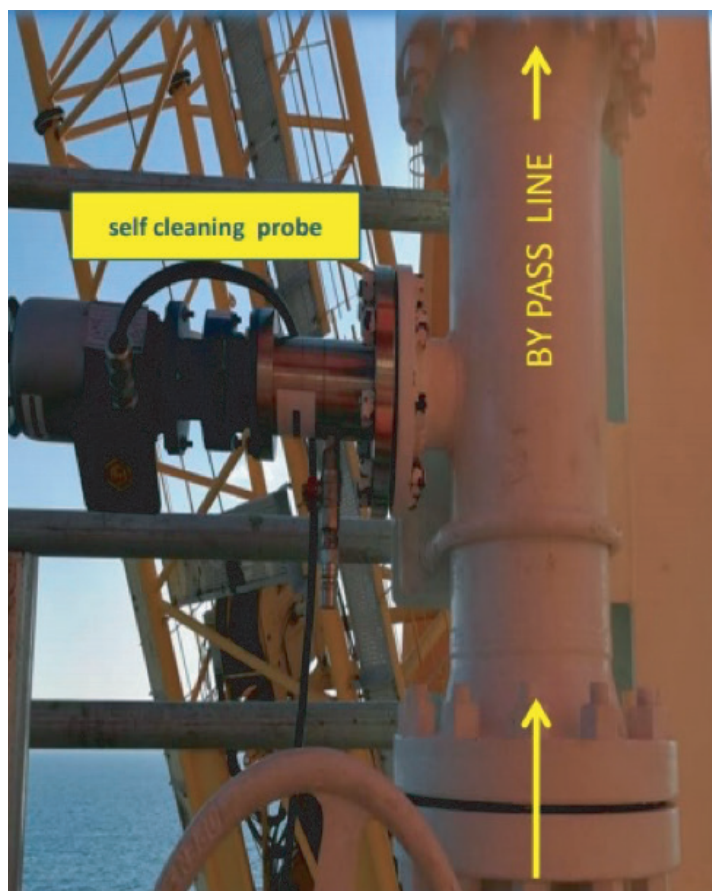
Fig.1: Self-cleaning probe installed on the 6" by-pass line
